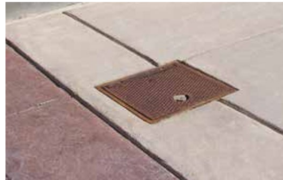
INSTALLED PHOTO, INGROUND HYDRANT TO BE INSTALLED IN SOD AREA
